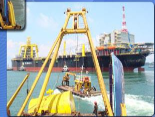
→ Unhooking Of Temporary Mooring System For Vessel FPSO P53
