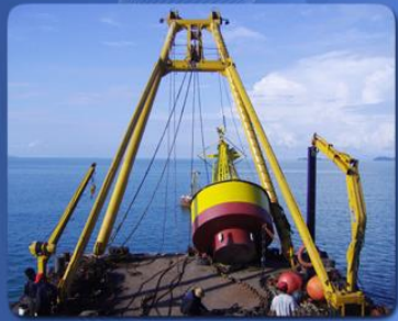
Laying Of Navigational Buoy At Indonesia - Batam
