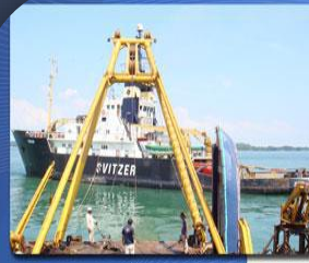
→ Hooking Up Of 6 Point Mooring System For FPSO Vessel - P53
