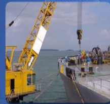
Heaving Up Port Side Anchor
