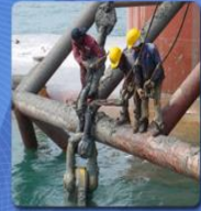
Rigging Up Lifting Wire For Anchor Replacement
