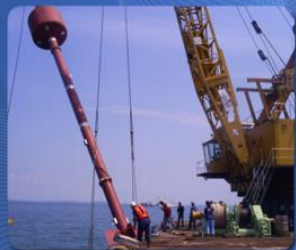
Installation Of Takong Resilient Light Beacon In The Singapore Straits
