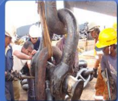
Installation Of 6 Point Mooring System
