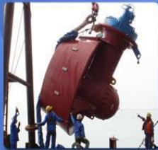
Lifting Of Thruster For Installation
