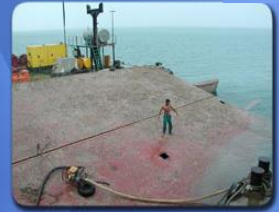
Upright Capsized Hopper Barge
