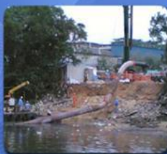
Inspection Of Pipeline Laying
